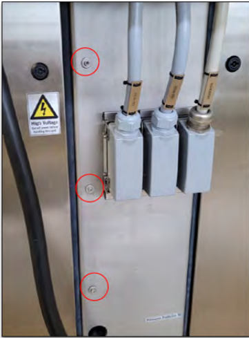
Figure 5 | Pre-drilled holes for EDM installation on GM24-48
