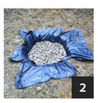
Line the hole with a permeable weed membrane (available at most DIY stores) and fill with scalpings, shingle or just crushed hardcore. The membrane will stop the hole silting up and allow water to collect and drain properly.
