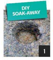
Dig a new hole at the bottom of the main hole about 2ft (60cms) in diameter and about 2ft (60cms) in depth.
