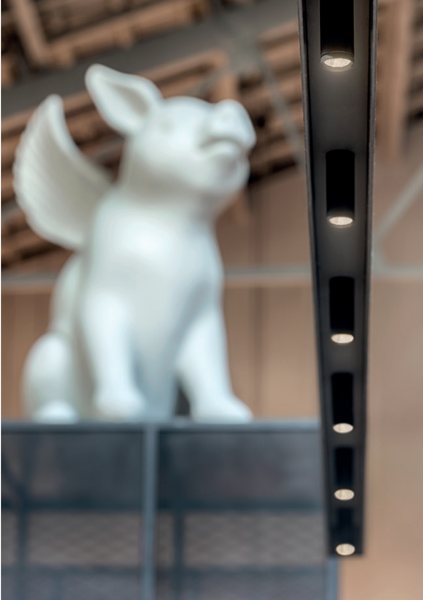
Note: Top installed in a long hollow suspended metallic piece.
