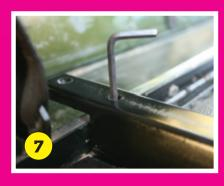
Use the long fixing bolts (50mm) at the front of the rails. This bolt passes all the way through the rail. Do not tighten this fixing fully at this stage.
