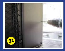
Fix into place using the smaller screw/rivet fasteners. These fasteners can also be tapped into place with a hammer.
