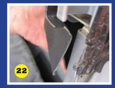
Trim the plastic with a sharp knife if necessary to achieve a snug, flush fit.
