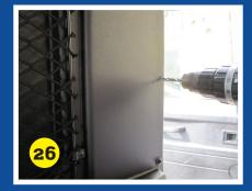
Fix into place using the smaller screw/rivet fasteners. These fasteners can also be tapped into place with a hammer.
