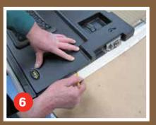
The longer pair of angled fixing plates fix to the lower portion of the door. Position the fixing plates to the inside of your pencil outline allowing for the thickness of the trim panel.
