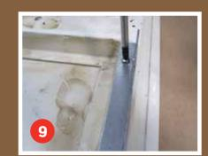
Repeat the process for the upper fixing points using the smaller of the angled mounting plates.
