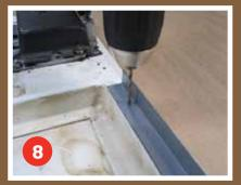
Fix the angled mounting brackets into the door frame using the stainless steel screws provided.
