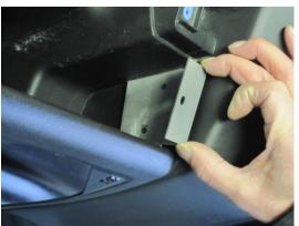
2. Drill the screw-holes for the fixings. Use a 3mm drill.
