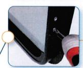
7) Remove the two screws at each end of the window frame.
