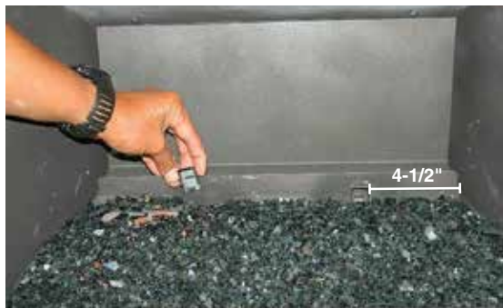
Log bracket install
