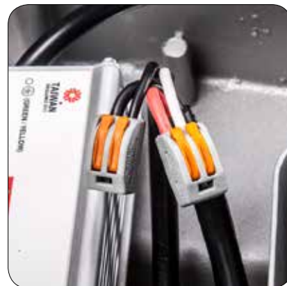
German WAGO® connectors for output wiring, safe and convenient
