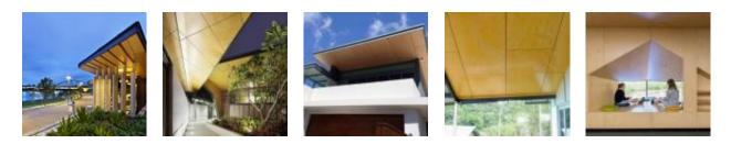
FacesA-CBondA-BondStress Grade F17EmissionsSuper E0StandardAS/NZS 2271 - 2004Core GapsSome (View example)Thicknesses1.5, 3, 4, 5, 6.5, 9.5, 12.5, 16, 19, 25, 32mmDimensions2400 x 1200, 2700 x 1200mm
