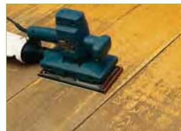
To renovate a floor, the lacquered surface must first be sanded down.
