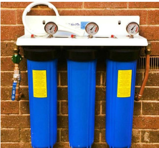
**9.** Check the housing for leaks and repair as necessary.
