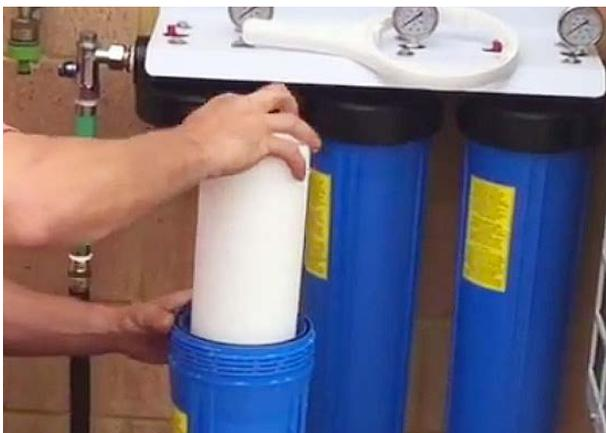
**6.** Install the new whole house big blue cartridges into the filter housings.
