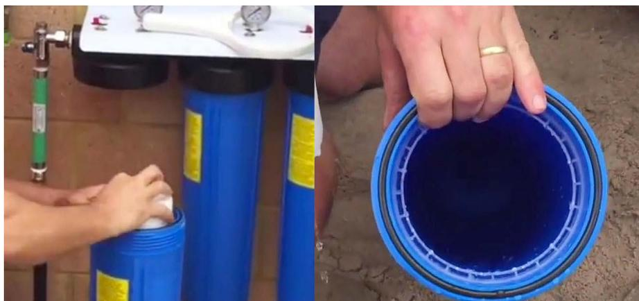
**7.** Ensure the cartridges center hole are seated in the stump in the base of each housing. Ensure the cartridge is centered & vertical as you lift the housing up into the head cap thread to replace. Hold 1 hand under the housing as you screw back on the whole house big blue filter housing by turning it clockwise. Do this until it is hand tight. If lubricated correctly this will screw on very easily without the tool.
