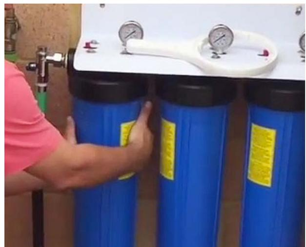
**5.** Remove the old filter and discard. Make sure to note the orientation of the cartridges.
