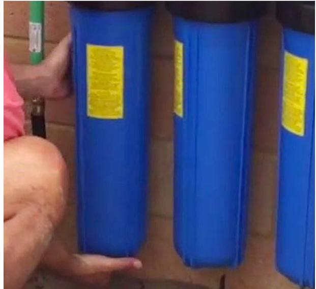
**8.** Insert the housing tool onto the filter housing. Tighten the filter housing until firm. Do not tighten until overtightened. Do not force.
