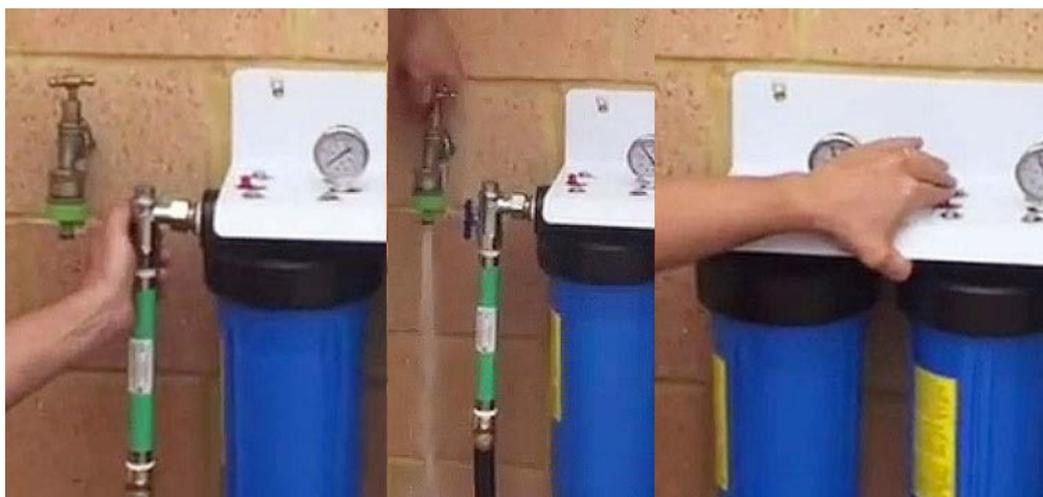
**12.** Turn off flushing tap. Turn on taps inside the home to release any air and you are done. Inspect the work area if there are no leaks etc and all is as it should be. Clean up.
