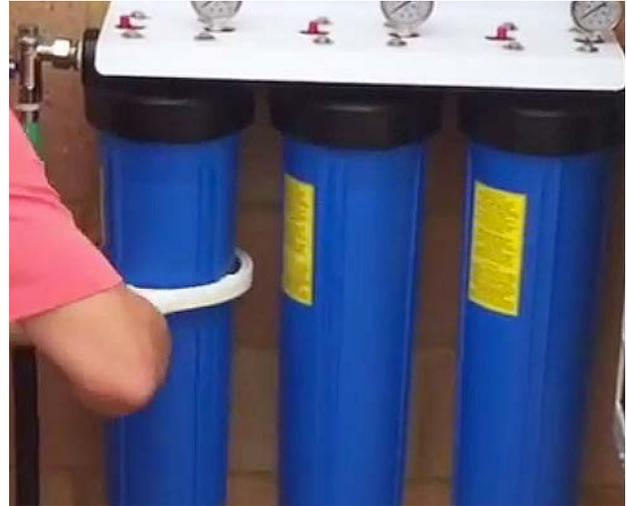
**4.** Once loosened with the tool, the housing can be removed by hand. Spin the housing counterclockwise. Spin until the housing is completely removed.
