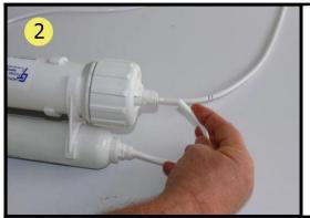
The pre-carbon and post-carbon filters will release some fines, we have left the line off before the membrane. When installed and ready for use, run water through the first filter until the water runs clear, then push the water line into the membrane housing firmly.
