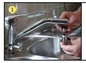
Screw off the aerator from the kitchen tap, then connect the diverter valve to kitchen mixer tap (using the adaptor provided, if required)
