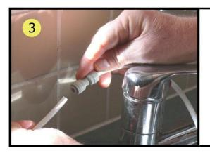
The diverter valve remains in place permanently. To disconnect or reconnect the filter, simply separate the water line at the inline joiner by depressing the outer collar on the joiner and pulling the water line out. To reinstall, simply push the line back in firmly.
