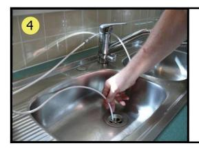
Reverse Osmosis Systems produces waste water, so place the drain line directly down the kitchen sink to dispose of this water
