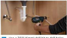
Use a 7/32" (6mm) drill bit to drill holes. Carefully tap the plastic anchors into the drilled hole with a hammer. Mount unit to the wall with the screws. Pull the protective plastic strip from the battery compartment. The red LED should flash and beep five (5) times to indicate that the battery is installed correctly.
