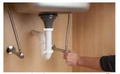
1 Unpack and unwrap contents. Turn off and disconnect the cold water supply.
