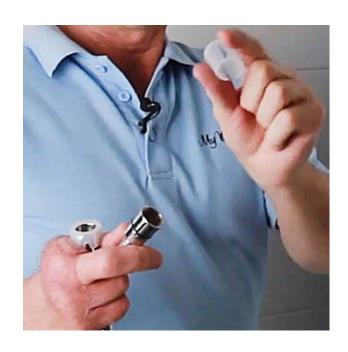
**7.** Insert the 1 x rubber washer into each shower hose end connector. This will prevent water from leaking out of the connector.
