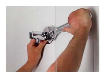
**5.** Use a tool or spanner to tighten firmly and secure in the right position, so the ½" male thread connection is pointing straight down.
