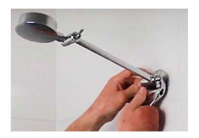
2. Make sure the shower supply pipe is clean and dry. If there are any old thread tape residues, take the thread tape off, then give it a wipe.
