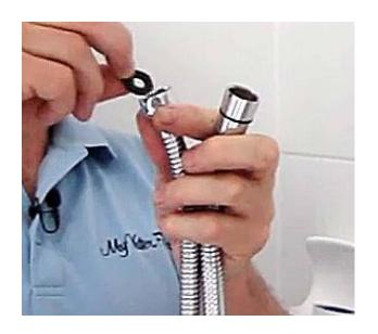
**8.** Attach the hexagonal hose end connector onto the ½" male thread connector of the shower bracket and hand tighten. Use a tool or a spanner to tighten firmly. Please do not overtighten as the rubber washer inside might get squashed and this will result with a water flow restriction. If there's leakage, you can apply thread tape to the ½" male thread of the shower bracket.
