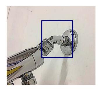
11. Once installed, hold an empty bucket under the shower head as you slowly turn the cold water on, allow the black colored carbon water to flow into the bucket until the black water turns clear again. Please note all carbon filters can emit black water from the carbon fines inside the filter when first used. Let it flow for a few seconds until the water has turned clear, adjust the temperature up to a normal shower temperature.
