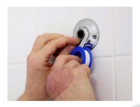
4. Screw the ½ inch female thread of the shower bracket holder onto the shower supply pipe on the wall and hand tighten. Please do not overtighten as the rubber washer inside might get squashed and this will result with a water flow restriction.
