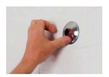
**3.** Wrap the thread tape in a clockwise direction around the shower supply pipe. Make sure to wrap it in the same direction, how you would screw your shower filter on to ensure you are not unwinding the thread tape as you screw on the shower filter. Avoid wrapping the center of the water pipe as that will block the hole. 6 full turns of thread tape should be sufficient.
