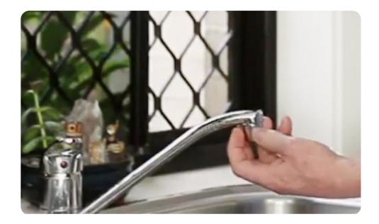
3. The diverter valve that comes with the system has a 21-millimeter female thread connection. If your faucet has a 21-millimeter male thread, ensure there is a rubber washer inside the diverter and simply connectby screwing the diverter valve straight onto your faucet thread.
