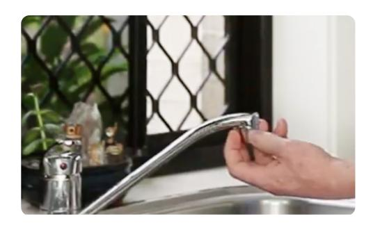
3. The diverter valve that comes with the system has a 21-millimeter female thread connection. If your faucet has a 21-millimeter male thread, ensure there is a rubber washer inside the diverter and simply connectby screwing the diverter valve straight onto your faucet thread.
