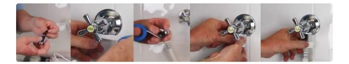
5. Wrap thread tape around the 1/4" male threaded end of the on/off ball valve.
