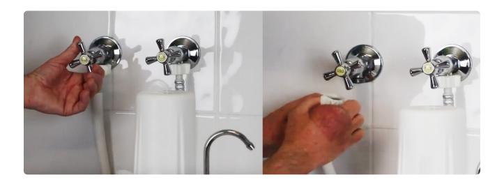
3. Unpack the <u>Easy Fit Laundry Connector 3/4" Male x 3/4" Female x 1/4"</u> Side Female Connection and ball valve.
