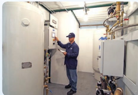
AS-J250-HPCR Containerized High Purity Packaged PSA Oxygen Plant for NATO Forces — Afghanistan
