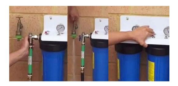
**12.** Turn off flushing tap. Turn on taps inside the home to release any air and you are done. Inspect the work area if there are no leaks etc and all is as it should be. Clean up.
