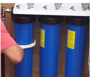
**4.** Once loosened with the tool, the housing can be removed by hand. Spin the housing counterclockwise. Spin until the housing is completely removed.
