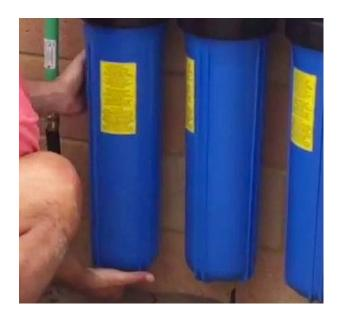
whole house big blue filter housing by turning it clockwise. Do this until it is hand tight. If lubricated correctly this will screw on very easily without the tool.
