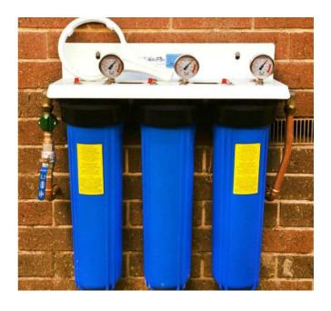
**9.** Check the housing for leaks and repair as necessary.
