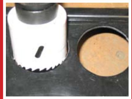
Cutting out the holes in the console is undoubtedly the time consuming part of the installation. Plan your layout carefully, take your time and don't rush it! How good a job you do of fitting the radio, switches and gauges etc will determine how well the finished installation looks. Importantly, always remember: *Measure Twice - Cut Once.*
