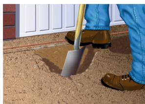
Dig trench 318mm wide (218mm wide if against a structure) by 278 mm deep for channel (483mm deep if installing sump unit). Mark finishing height with fixed line 3mm below final surface. Lay 100mm (min.) bed of C14/15 concrete.
