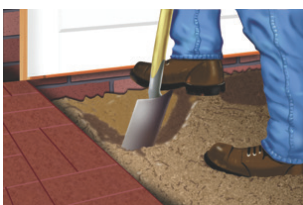
Dig trench 100mm wide by 210mm deep for channel. Remove cap from outlet.
