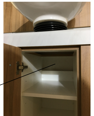
Plumbing void to rear of cupboard
