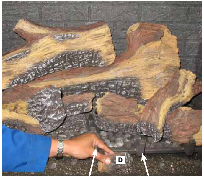
Burner Grate Post 3
