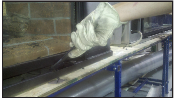
Figure 11.3. Inserting Glass Clip Tool
