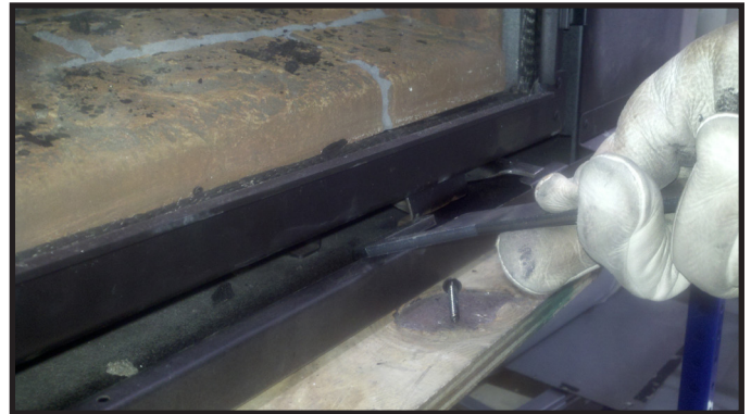
Figure 11.2. Glass Clip Tool Location
