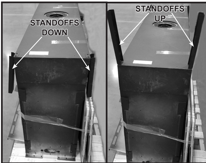
Standoff Shipping Position Standoff Installation Position
