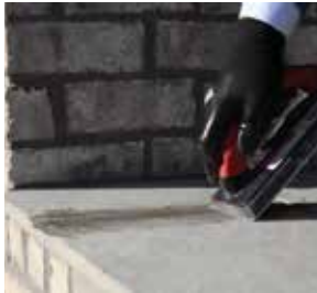
PIC 1. Fill joint with grout.
