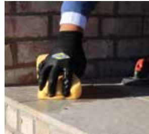
PIC 2. Remove excess grout with clean water.
