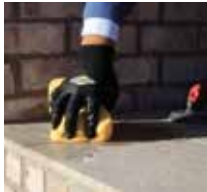
PIC 2. Remove excess grout with clean water.
