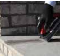
PIC 1. Fill joint with grout.
