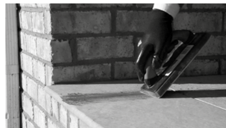
PIC 1. Fill joint with grout.
