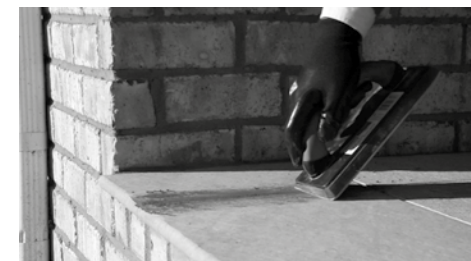
PIC 2. Remove excess grout with clean water.
