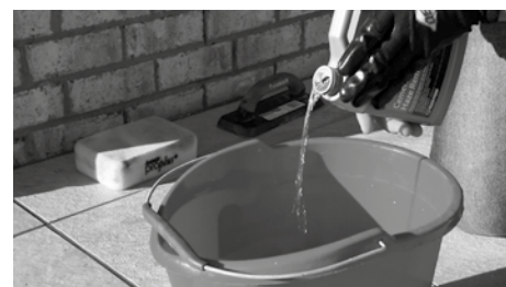
PIC 3. Add specific acid cleaning agent for porcelain tile to clean water.
