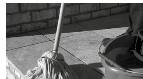
PIC 4. First floor deep cleaning after 12/48 h from installation.
