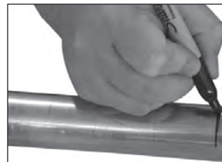
Figure 3 — Marking for Insertion Depth
