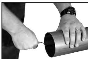
Figure 3: Deburr inside diameter deburring tool
