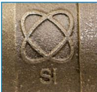
**NIBCO® HydraPure® valves can be identified by the double oval symbol and "Si" – indicative of silicon Performance Bronze® – cast in the body of the valve.**
