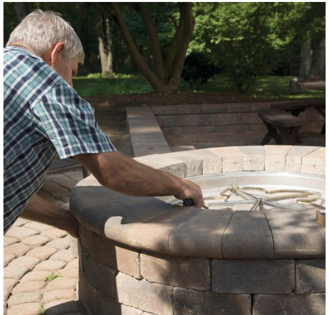
Figure 9.1 – Match-Lit test start-up
