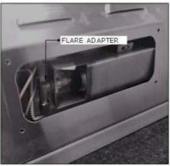
**11. Remove Brass O-Ring to Release Flare** Once the flare is removed, pull the orifice end out so it is accessible.
