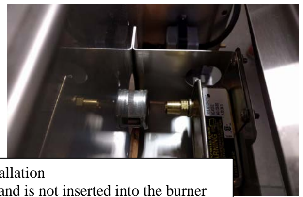
Correct installation The gas valve orifice is completely inserted inside the venturi
