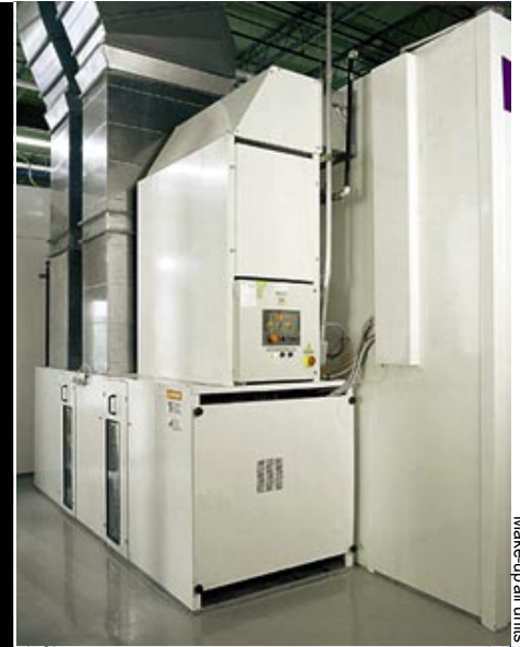
Make-up air units
