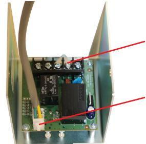
Connect all boiler wires per IOM. (In some cases it may require running neutral wire. Control requires constant power to operate).
