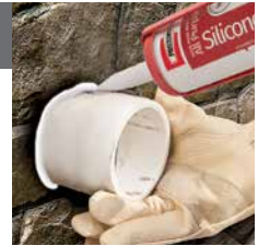
Caulk wall opening.
