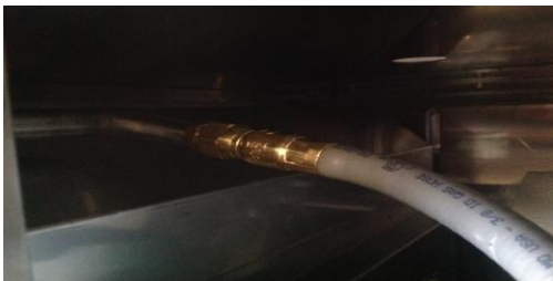
LP HOSE AND REGULATOR CONNECTION TO MANIFOLD
