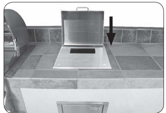
Fig. 3-2 Drop unit into place
