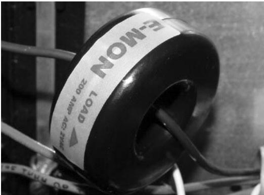
**Fig. 6. Solid Core Sensor Assembly.**
