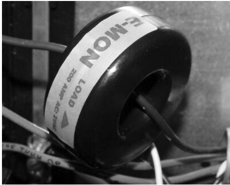
Fig. 6. Solid-core Current Sensor.
