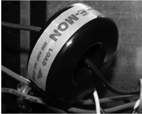
Fig. 6. Solid-core Current Sensor
