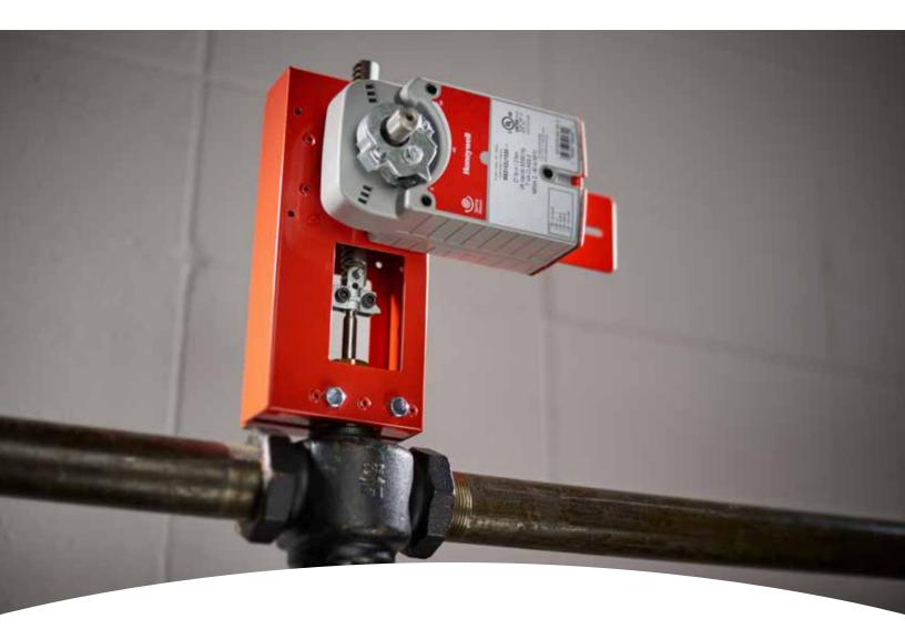
The new Honeywell Q5024 linkages enable retrofitting globe valves with Honeywell's leading direct coupled actuators (DCAs).
