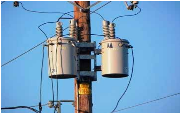
Open Delta (Wire Connection)
