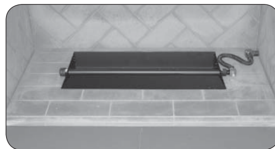
Fig. 11-2 Center burner in fireplace
