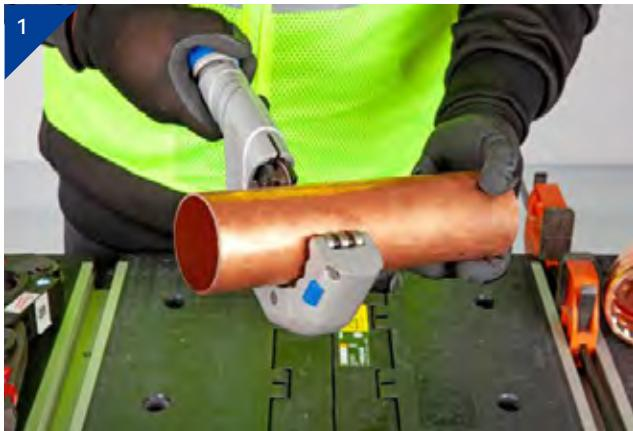
1. Cut copper tube to length using a pipe cutter or fine tooth saw and ensure the pipe is cut square.
