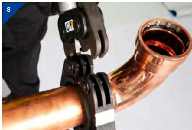
8. Select the adaptor jaw, insert onto the pressing tool and arrest the locking bolts of the tool.
