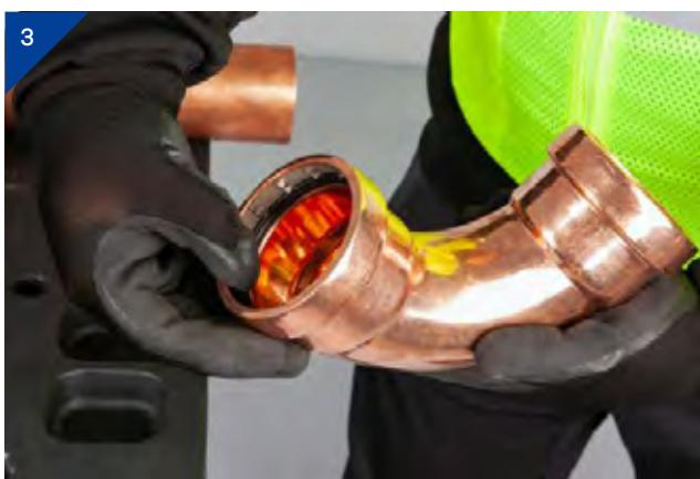
3. Ensure you have the correct sized fitting, check the fitting is clean and the stainless steel grip ring and O-ring are free from debris and correctly seated in the fitting.
