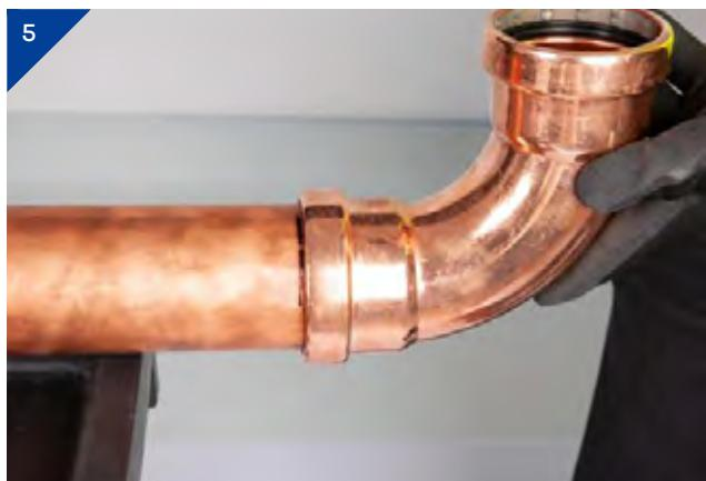
5. Secure the tube in a vise or pipe support to prevent any movement of the tube and insert the fitting onto the tube. Ensure the outer edge of the fitting lines up with the insertion depth mark made in step 4.
