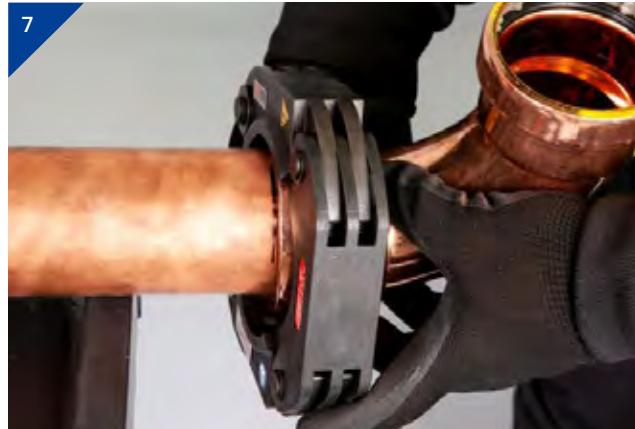
7. Open the collar and place it around the fitting, such that the bump on the fitting is rested into the groove of the pressing collar. Close the press collar ensuring it fits square with the fitting and check the insertion depth mark still lines up with the outer edge of the fitting.
