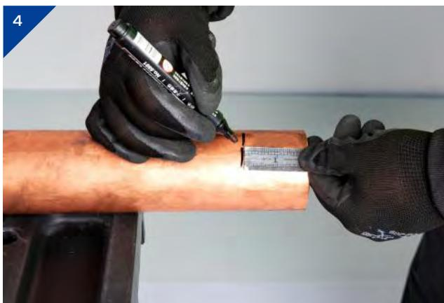
4. Measure insertion depth with ruler. Then mark the proper insertion depth on the outside of the tube.
