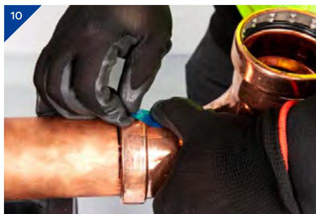
10. Release the adaptor jaw from the collar and the collar from the fitting. Remove the label to indicate completion of the press.
